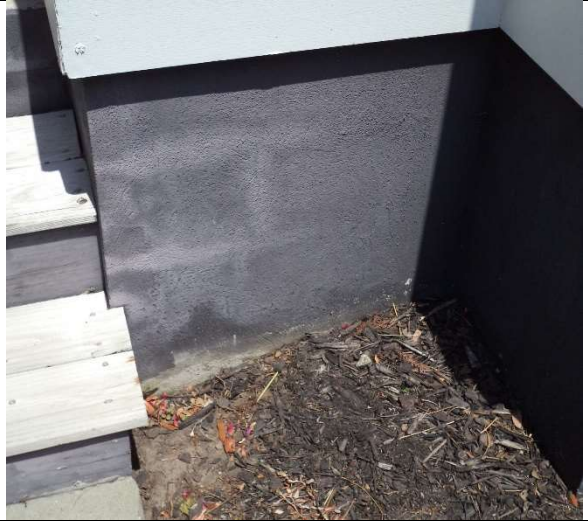
Block Wall Foundation (Typical)
