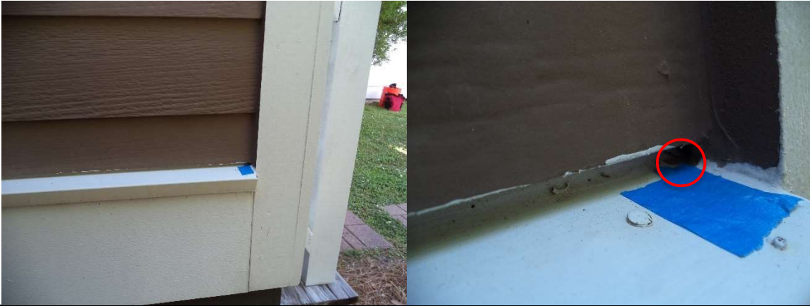
Rear Porch – Small hole for insects to penetrate to wood
