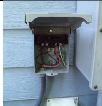
HVAC Fused Disconnect at external unit
