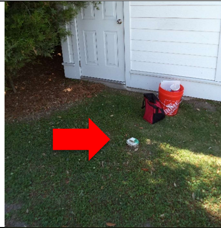
Sanitary Sewer Cleanout – presumed Secondary
