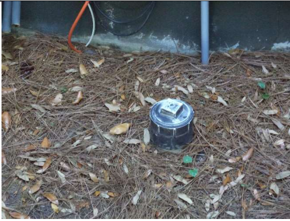
4" PVC Sanitary Cleanout – presumed Primary
