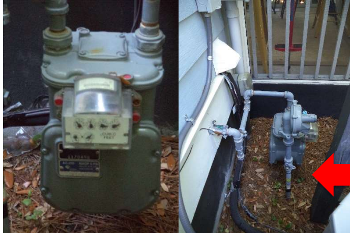
Gas Meter and Shutoff valve
