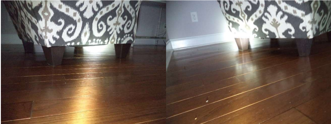
Living Room Flooring presumed to be installed over vapor barrier on top of concrete slab
