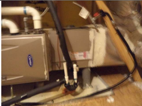
Furnace Gas Shutoff Valve and Supply line
