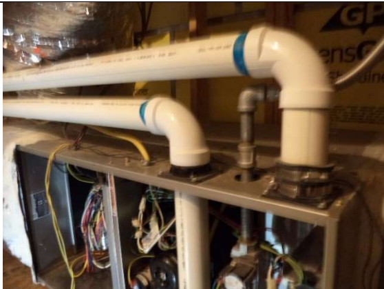
AHU w/o Cover and Intake/Exhaust Piping
