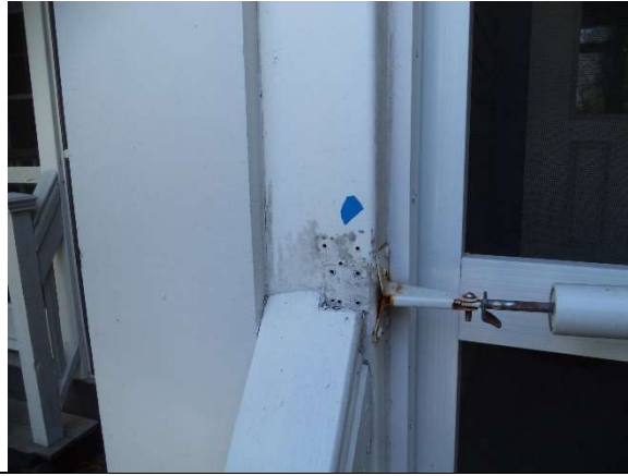
Rear – Porch Screen Door hydraulic cleat attachment holes
