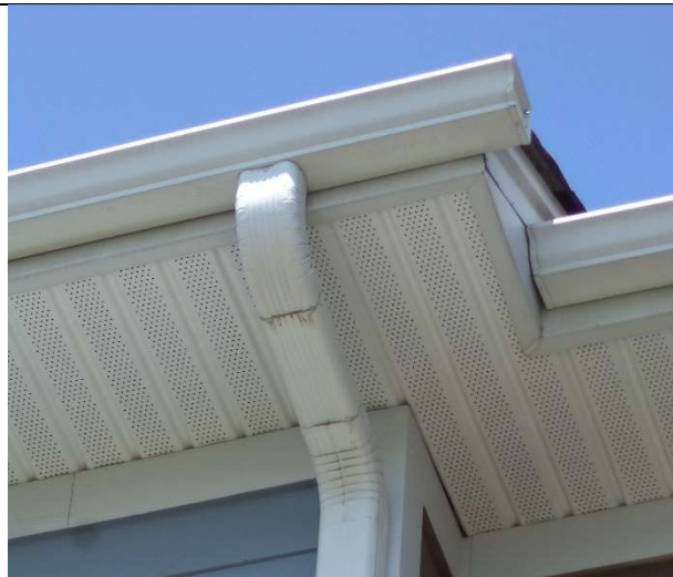
Roof Ventilation – Soffit Vent (Typical)
