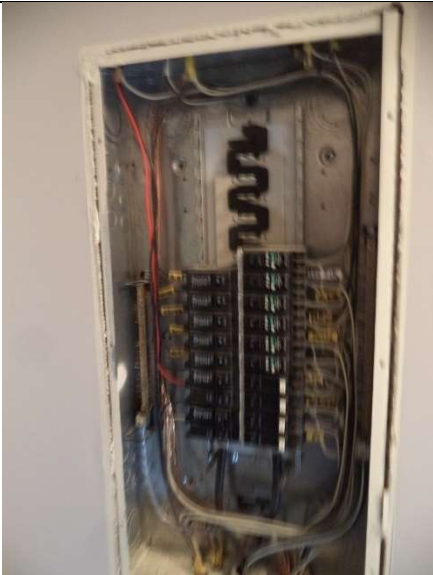
Eaton Distribution Panel with AFCI/GFCI CKT BKR
