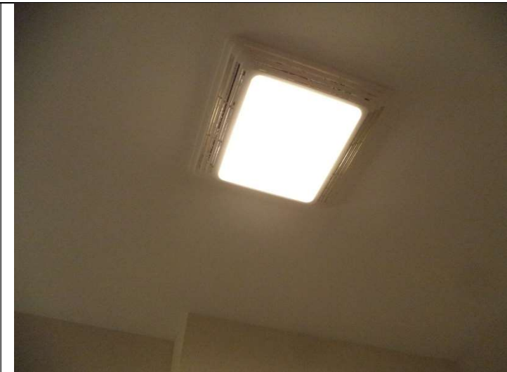
Bathroom Fan w. Light operating by wall switch (typ)
