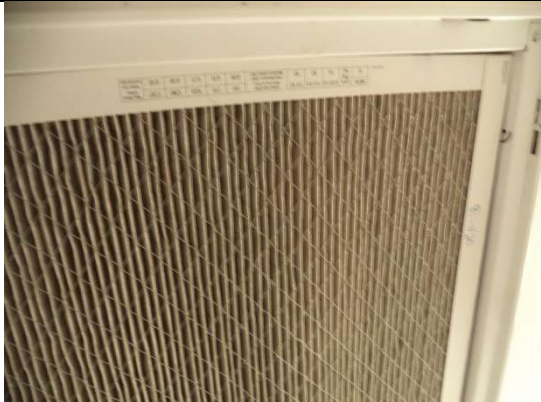
2 nd Floor – Air Return Filter
