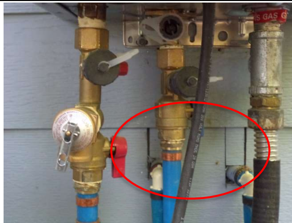
Rear – Instantaneous HW penetrations in siding
