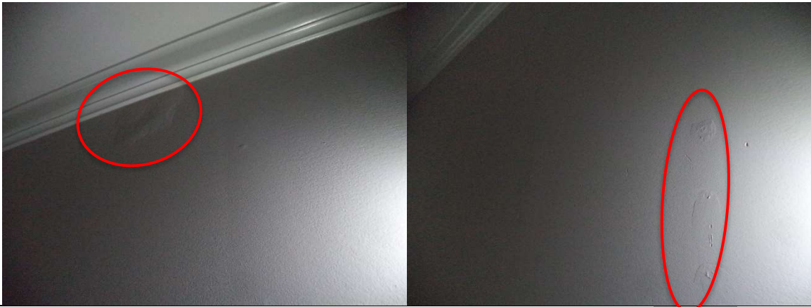
Living room - Indeterminate Patch | wall repair – nail/screw holes
