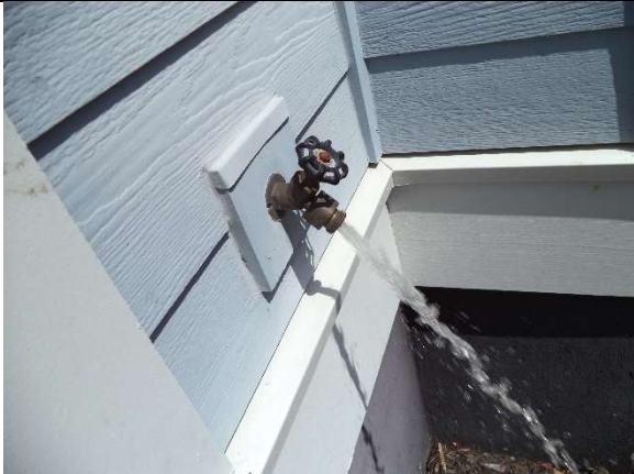
Front - Hose bibb with vaccum breaker
