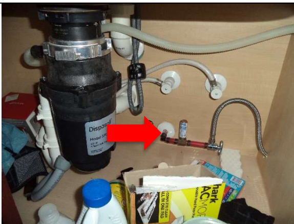
Dishwasher supply – 1/2" PEX to SS Braid Hose
