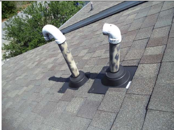
Furnace Air Intake and Exhaust Flue
