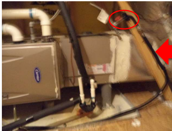
Furnace Shutoff Valve circled | CSST Hose indicated by arrow | Care should be taken when placing any personal items in the attic to prevent damage to the gas supply
