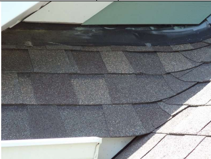
Roof Flashing (Typical)
