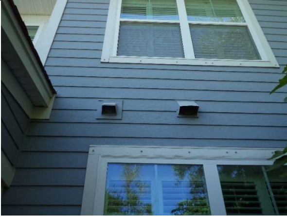
Dryer Exhaust Vent
