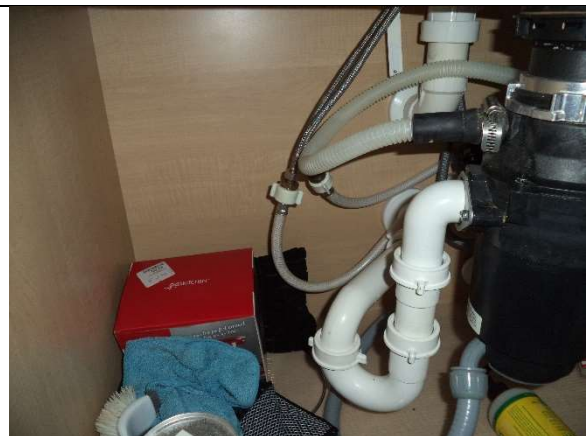
Under Kitchen Sink Supply and Drain
