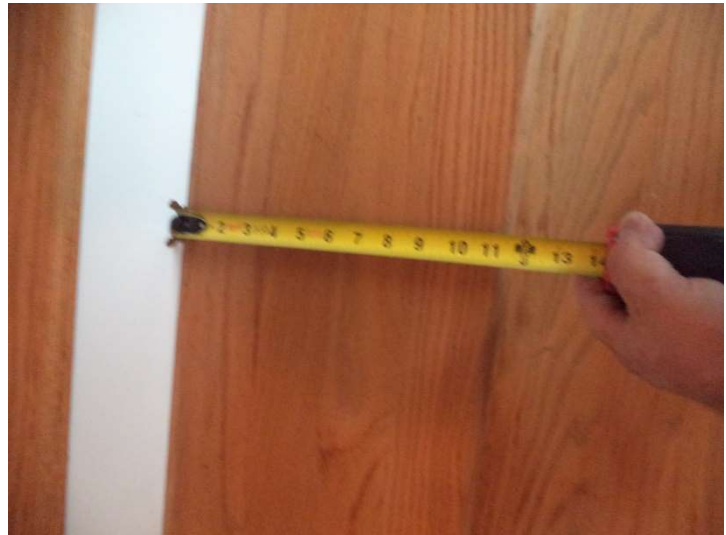
Stair tread shall be no less than 10" run and 7 \frac{3}{4} " Rise" | Shown are 11" run and 6 \frac{3}{4} " rise
