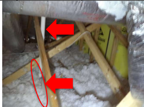
Bathroom Stack Vent – 1 1/2" PVC
