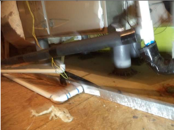
Condensate Line | Secondary Line | Drip Pan
