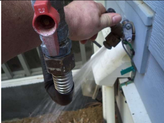
Rear - Hose bibb with vaccum breaker
