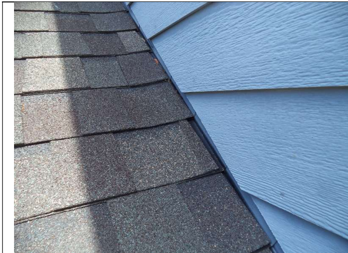
Roof Flashing (Typical)
