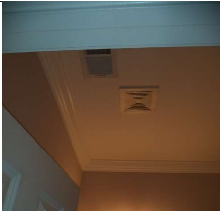
1 st Floor Air Diffuser and bathroom exhaust fan
