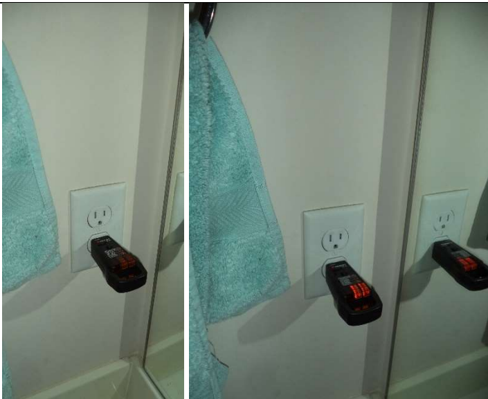
Bathroom GFCI trip tested and reset (typ)
