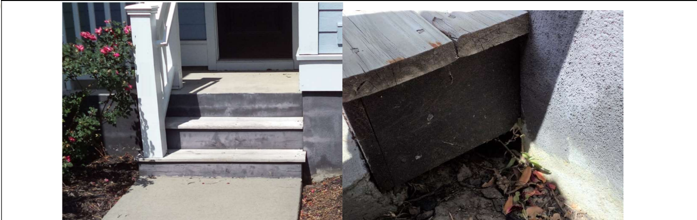
Front Stair | Hole below stairs should be filled to prevent water and wildlife
