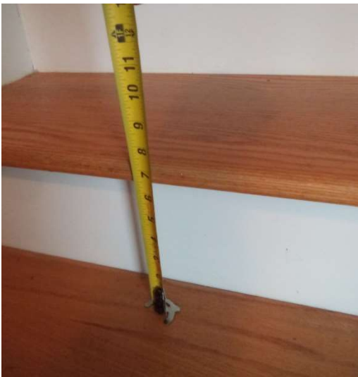
Stair tread shall be no less than 10" run and 7 \frac{3}{4} " Rise" | Shown are 11" run and 6 \frac{3}{4} " rise
