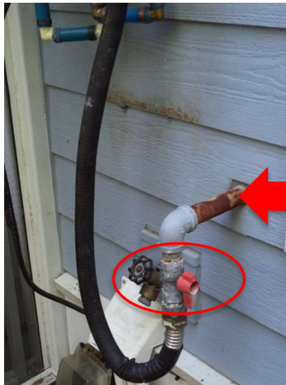
Rinnai HW HTR Shutoff Valve circled | Galv. Steel supply should be coated to prevent potential for leaks at threading or pinholes
