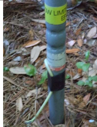
Gas Supply with locator wire
