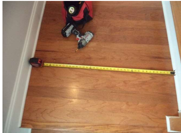
Stairway width shall be a minimum of 36" | Shown is ~ 40" for landing and stair
