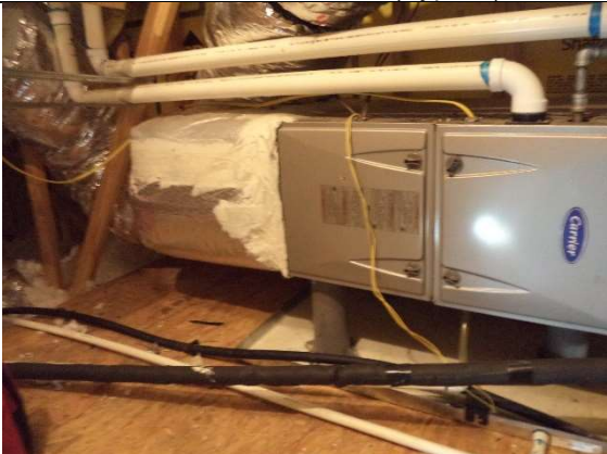
Attic - Carrier AHU and Gas Furnace
