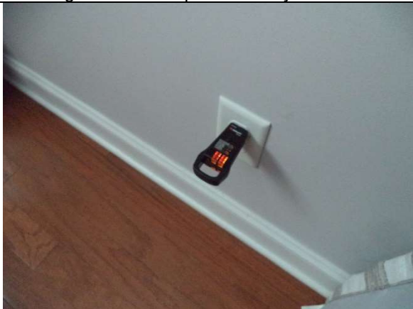
Interior outlets indicating correct function (typ)
