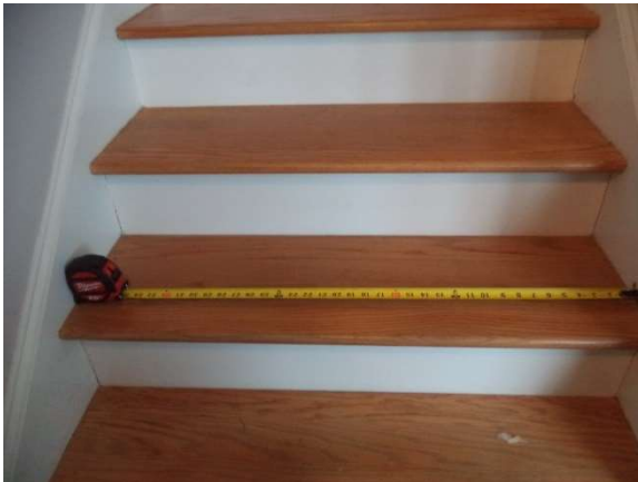
Stairway width shall be a minimum of 36" | Shown is ~ 40" for landing and stair
