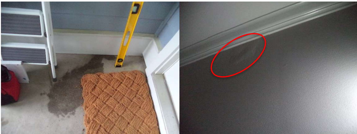
Stain on Porch Concrete and Upper Drywall Repair
