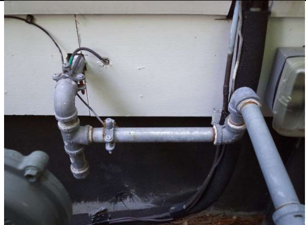
Rear - Bonded Gas Supply Entry to Home
